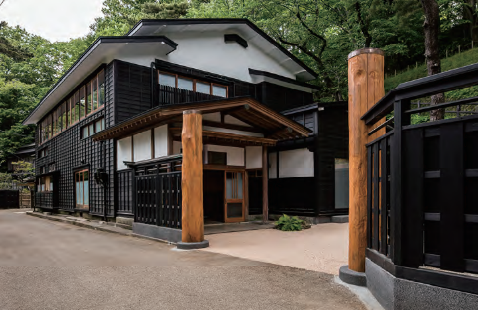
Fig. 14 Renovated Historical Building "Akita Culture and Industry Facility Matsushita"
